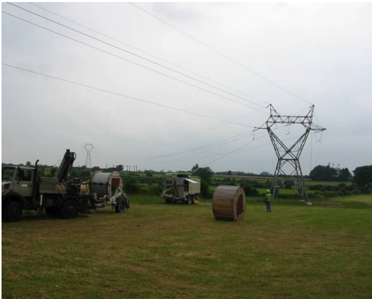
Illustration 5.9: Stringing location during operation.
