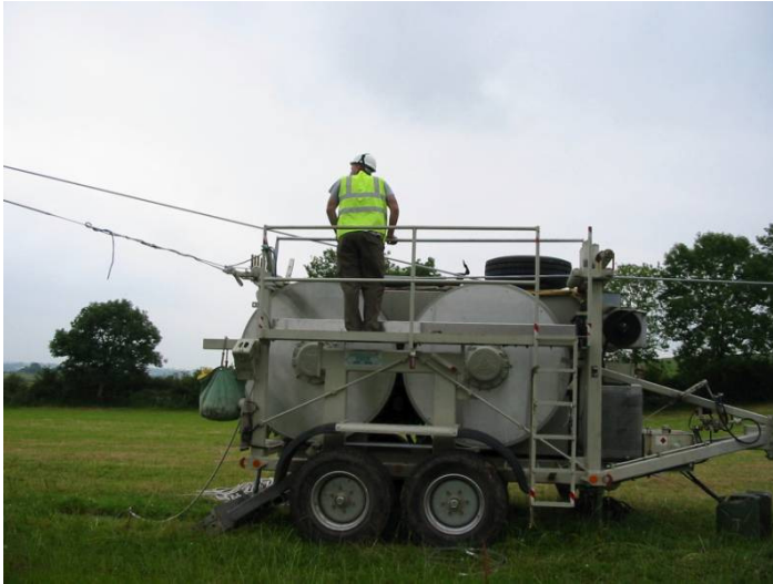
Illustration 5.8: Winching machine for stringing operation.
